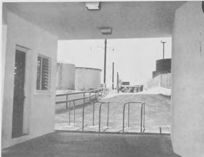
LAGO'S NEW refinery entrance will go into operation Tuesday morning, June 4. This photo was taken looking through the covered walkway toward the Main Gate. Time card racks will be installed on the curved wall, right. Lago police will occupy the enclosure on the left; government police, the enclosure behind it.
